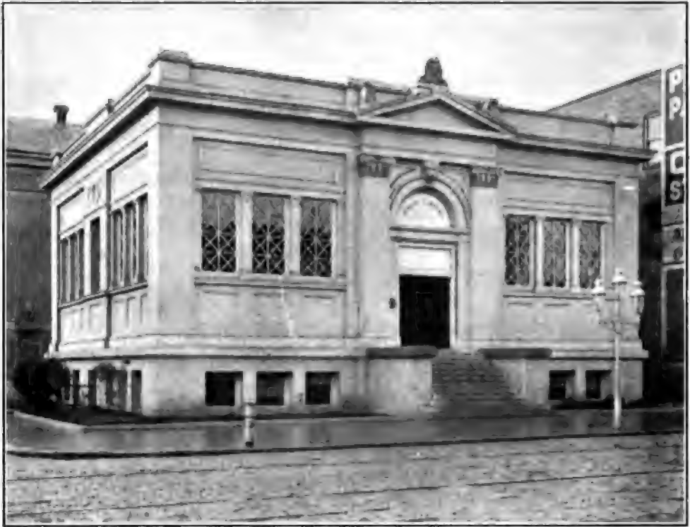
BRANCH LIBRARY NO. 5, FOURTH AND CLARK STREETS: PRESENTED BY JAMES D. PHELAN Street, photo
